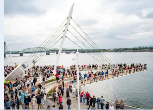
Grant Street Pier & Waterfront Park
